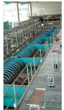
Courtesy Photo: Siemens
